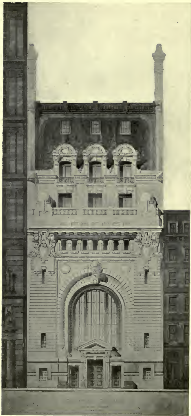
THE NATIONAL PARK BANK. (Broadway Façade.)
